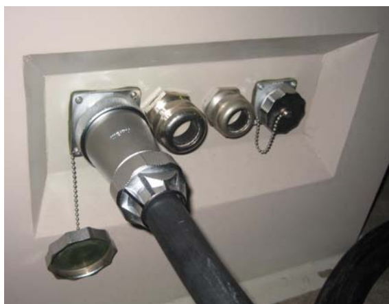
Cable Connection - by Plug and Socket. - quick connection.
